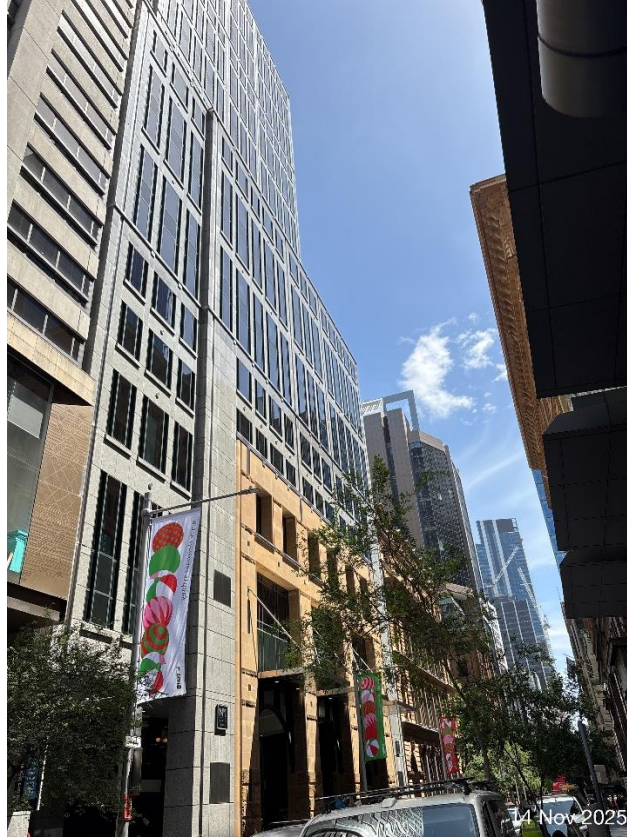
Figure 1: 1 Martin Place, Sydney, viewed from the east.
